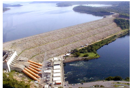
Akuse Hydroelectric Dam
